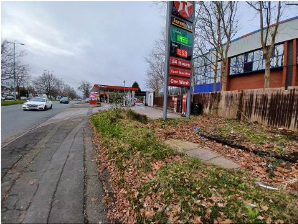
View south with Kingsway to the left and the Petrol filling station centre with the existing B and M store to the right
